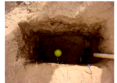
Backfill to 4 ft & place marker
