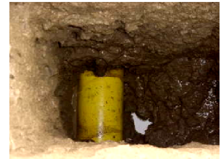
Expose Facility at 7 ft depth
