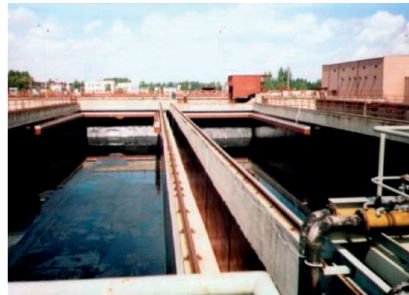
Waste water Reservoirs
